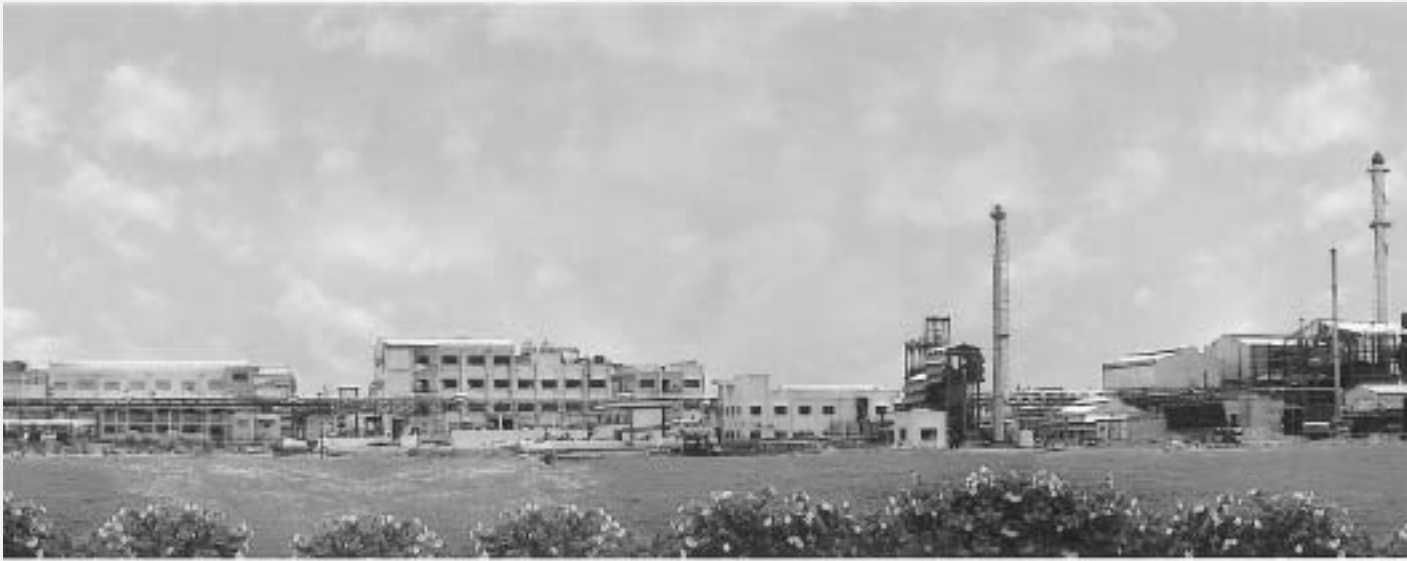
A bird's eye view of the Pydhibhimavaram Unit
