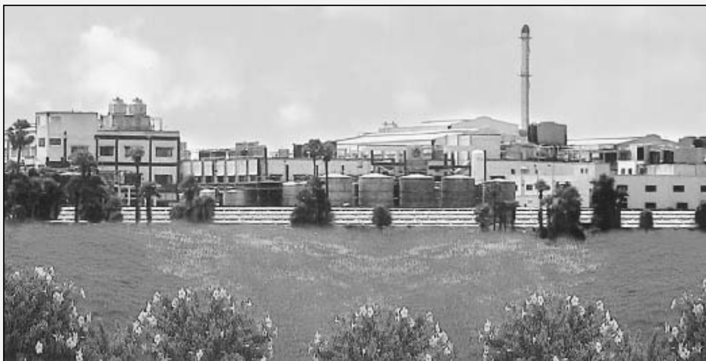
A view of the Pydhibhimavaram Unit
